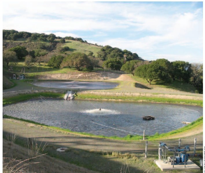
Ponds are among the simplest of biological treatment systems in that they rely on low, native concentrations of bacteria to accomplish treatment.
