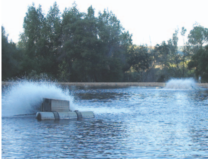
Selection of an aeration device represents the largest single equipment and operating expense associated with pond treatment. Above: Floating brush aerators in use at The Hess Collection Winery.
